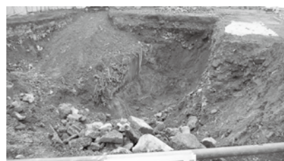
▲旧IRD焼却炉撤去跡
